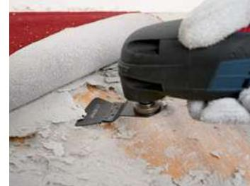
**Restos blandos de pegamento, moqueta, material aglutinante, material de juntas, silicona...****Soft remains of glue, carpet, agglutinative material, joint-material, silicone...****Copeaux tendres de colle, tapis, matière aglutinantes, matériel de jointes, ...**
